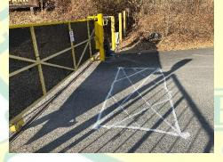
that was being activated by the sunlight causing the gate to lock open. When the gate company arrived to diagnose the issue, it turned out the problem was the in- ground sensor getting triggered as the asphalt heated up.
